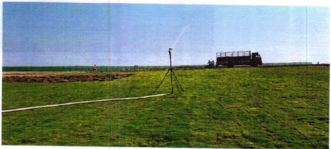
Permeate used for watering green cover on top of capped dump
