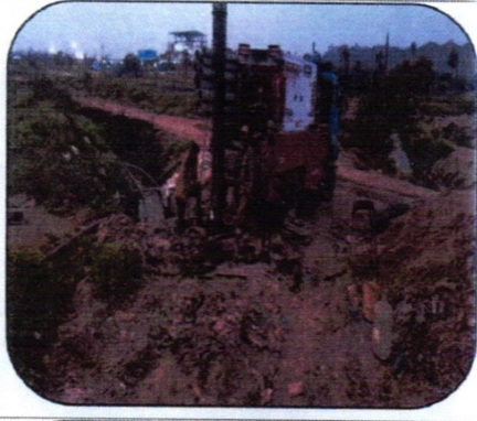
BW - 05 17°31'26.9"N, 78°35'45.7"E (Near SLF RCC Sump)
