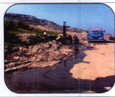
BW - 02 17°31'32.4"N, 78°35'25.7"E (Malkaram DG Room)
