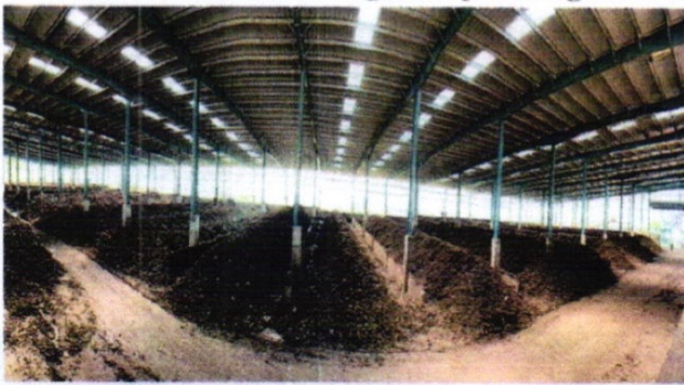
Windrows in closed PEB shed
