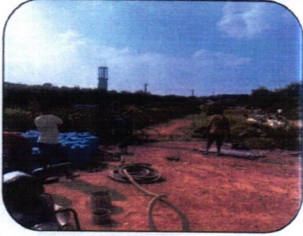
BW - 06 17°31'17.2"N, 78°35'51.0"E (RCC Flush Pond)
