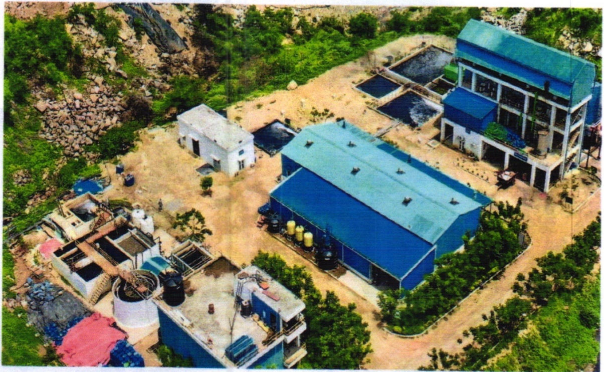
Waste Water Complex: Pre-treatment, RO shed, MEE-ATFD system (left to right)
